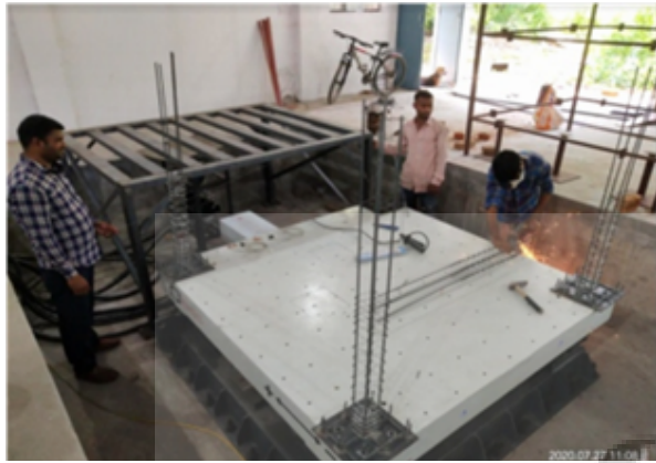
Installation of Large Shake Table
