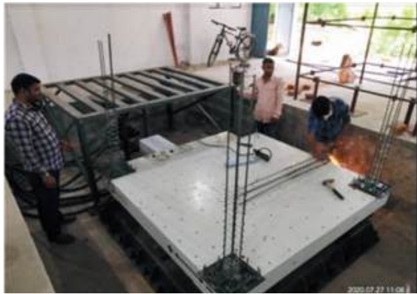
Installation of Large Shake Table
