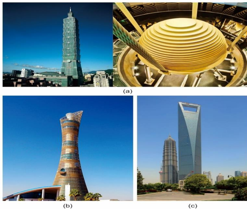
Figure 3. Tuned mass damper applications: (a) 101-Taipei, Taipei—Taiwan; (b) Aspire Tower, Doha—Qatar; (c) Sanghai World Financial Center
